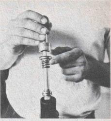
Install replacement cylinder. Note location of coil spring around cylinder. This is an anti-foaming device and must be in place at the approximate center of cylinder.
