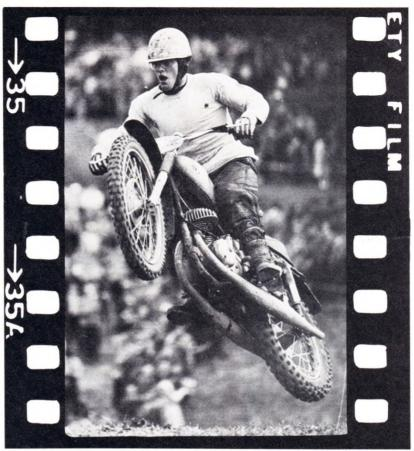
Production twin-pipe CZs sold much better after the Europeans' first successful tour of the U.S. Note that the carburetor feeds into the crankcase casting rather than the cylinder. Even way back when this model was around, the CZ transmission was building up a great reputation.
